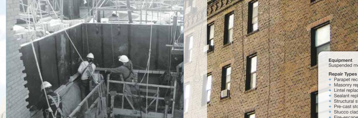
Suspended modular scaffolding using outrigger beams
